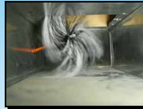
STEP 9 BONUS!!! WE BRUSH THE TRUNK LINES WITH A MOTOR DRIVEN ROTARY BRUSH.
