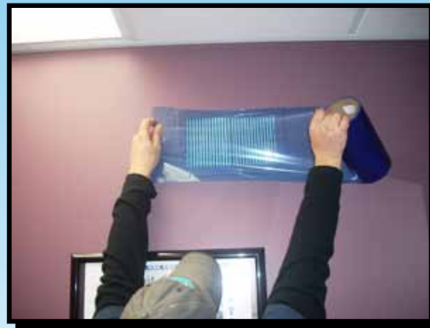
STEP 7 REGISTERS ARE COVERED TO TRAP DIRT AND INCREASE VACUUM PRESSURE.
