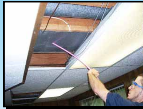
STEP 8 CLEAN THE DUCTWORK USING VARIOUS BRUSHES AND CLEANING TOOLS.
