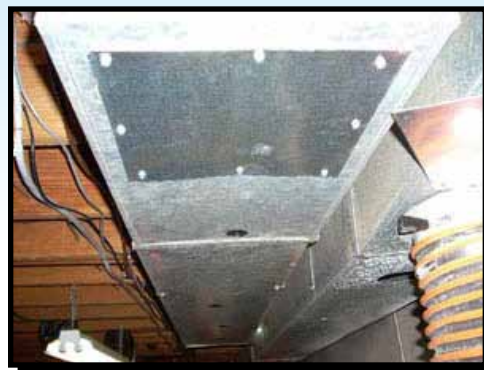
STEP 12 TECHNICIAN SEALS ACCESS OPENINGS AND RETURN SYSTEM TO SERVICE.
