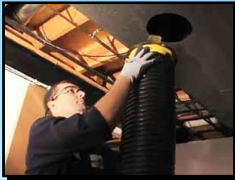
STEP 6 ACCESS OPENINGS ARE CREATED FOR OUR VARIOUS CLEANING TOOLS.
