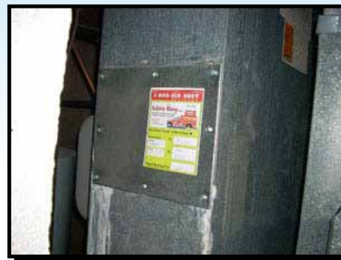
STEP 13 TECHNICIAN CLEANS AREA & PLACES A REMINDER STICKER ON THE FURNACE.
