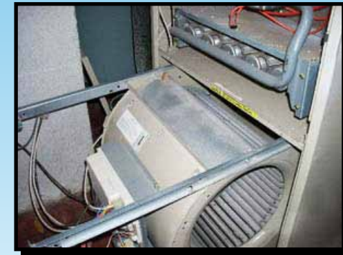
STEP 10 WE CLEAN YOUR FURNACE BLOWER, THE HEART OF YOUR FORCED AIR SYSTEM.
